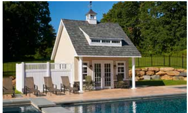
Heritage Liberty Pool House / 16' x 14' Special Siding, White Trim, Special Shingles Options Shown: 1 Extra 24" x 36" Window, 2 Extra Transom Windows, Stucco Exterior Upgrade, Stone Veneer (Special), 24" Carlise Cupola, 12/12 Roof Pitch, 3 Transom Mini Dormer
