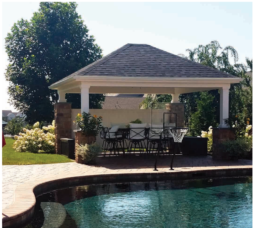
14x16 Vintage Pavilion privacy wall stone footers
