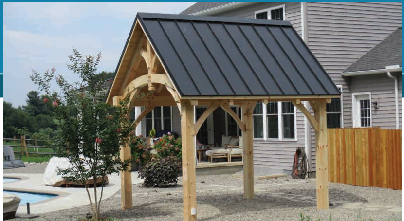
10x12 Timberframe Pavilion standing seam metal roof
