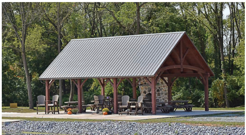
20x32 Timberframe Pavilion fireplace metal roof special stain
