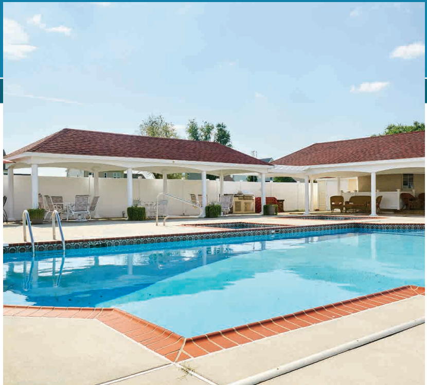
15x36 Vintage Pavilion electrical package attached 10x11 vinyl pergola
