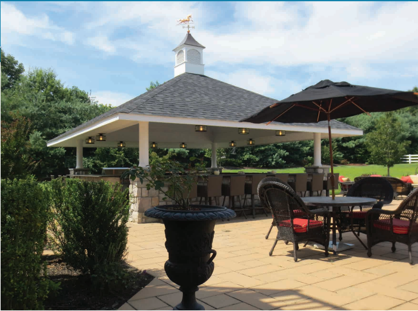
20x20 Custom Pavilion outdoor kitchen electrical package cupola
